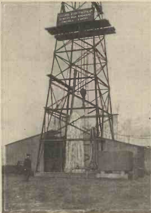
Showing water issuing from a boring.
