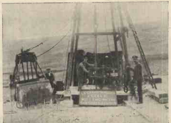
Boring operations in progress.
