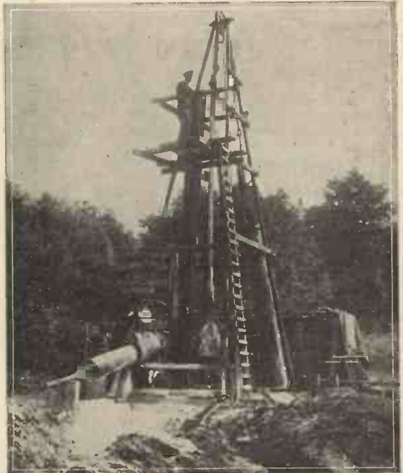
An 18-in. borehole at Sheringham which yields 12,000 gallons per hour.
