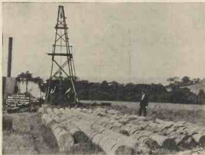
This photograph shows a number of 16-in. cores obtained from a boring 1,152 ft. deep.
