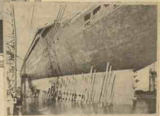
Fig. 3.—The photographs show clearly the launching plate, fire poppets and hydraulic rams.
