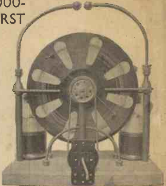
Figs. 1 and 2.—Front and back views of the Wimshurst Machine described.
