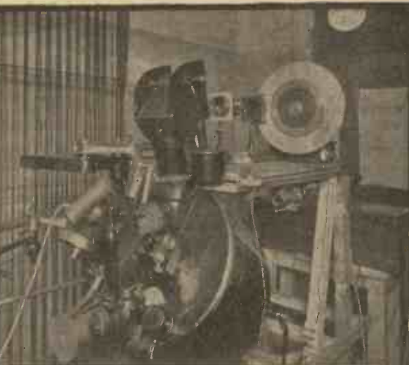
Fig. 2 (Left).—One of the original Arcadia projectors used for televising talking films in the early days. (Continued on page 389.)
