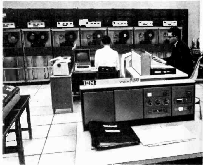
Magnetic data storage machines and information input and access points, in use inside the computer room, are shown above, whilst below an engineer is shown setting up one of the three IBM computers which form the main brain of BOADICEA
