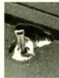
A "dry" joint. Solder failed to flow.
