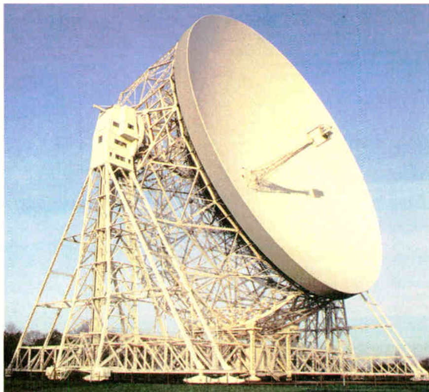
The dish of the Lovell telescope at Jodrell Bank weighs 1500 tonnes. (Photo: Ian Morison)
