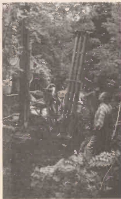
Borehole drilling at Poole's Cavern.
