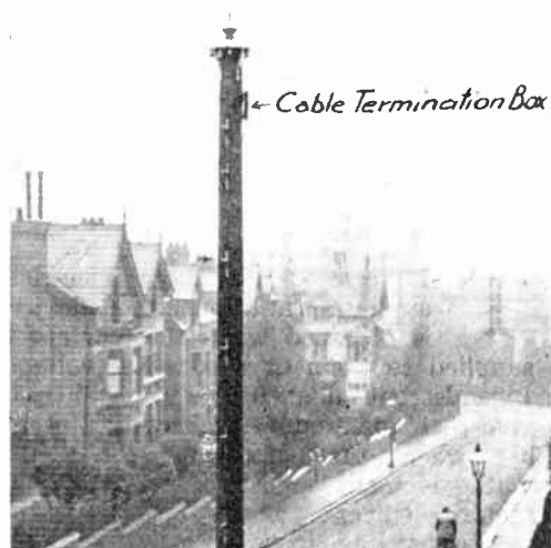
Fig. 36.—NEW TYPE OF POLE FOR TAKING WIRES TO SUBSCRIBERS' PREMISES.
