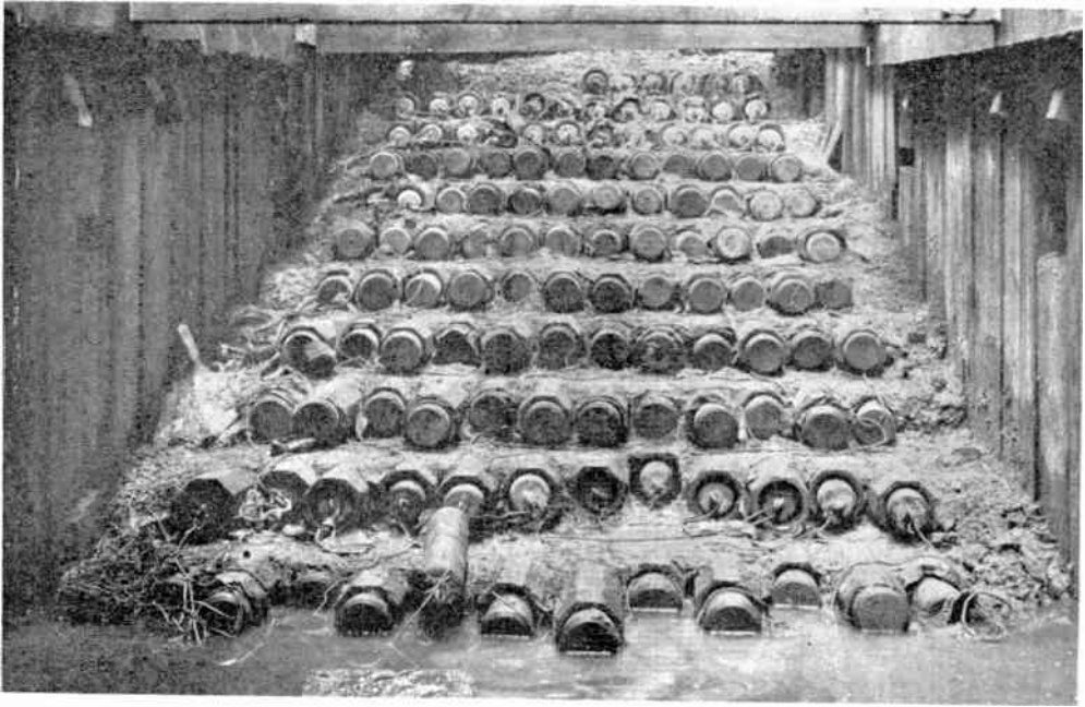
Fig. 32. —LARGE DUCT ROUTE UNDER CONSTRUCTION.
