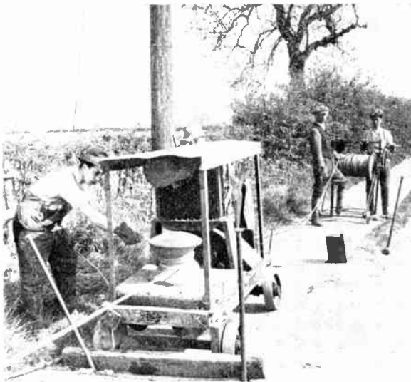
Fig. 35.—PULLING-IN A CABLE.
