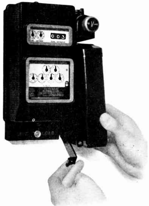
Fig. 9.—PREPAYMENT METER (FERRANTI) WITH EXTERNAL PREPAYMENT ATTACHMENT AND COIN BOX.
