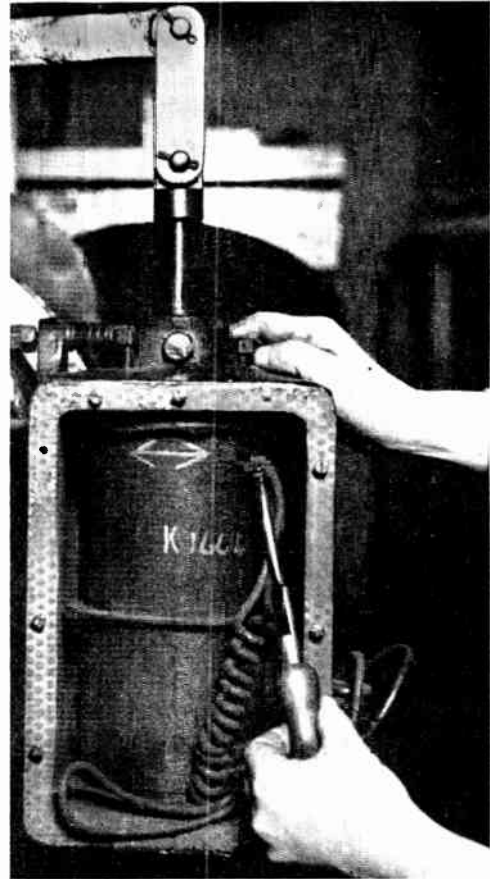
Fig. 25.—OVERHAULING THE CONNECTIONS TO THE MAGNET WINDINGS OF A SOLENOID "BRAKE" WHICH ACTS ON THE SHAFT OF A MOTOR.
