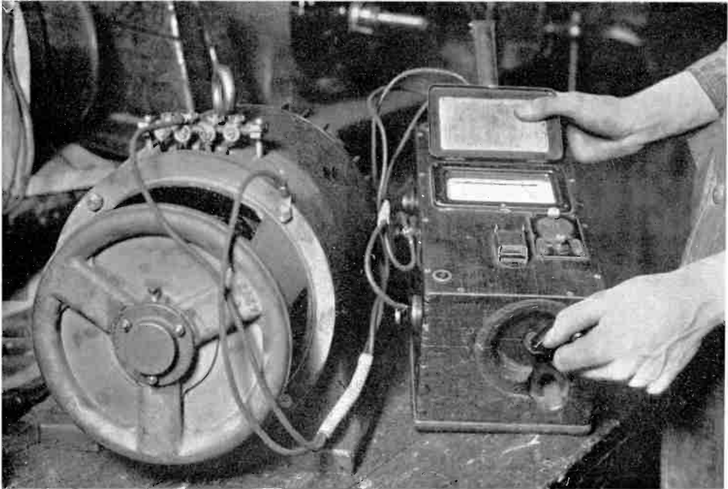
Fig.10.—TESTING WITH A MEGGER FOR LEAKAGE FROM WINDINGS TO FRAME. ( Lancashire Dynamo and Crypto, Ltd. ) The megger voltage should be at least twice that of the machine under test.
