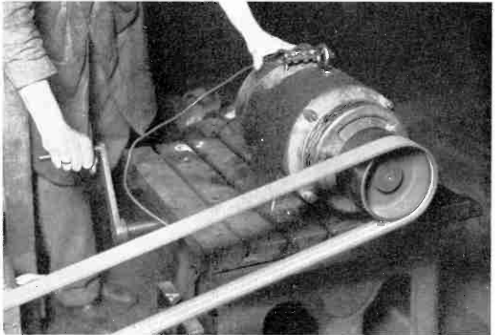
Fig. 4.—ADJUSTING BELT ON TEST BENCH. ( Lancashire Dynamo and Crypto, Ltd. )
