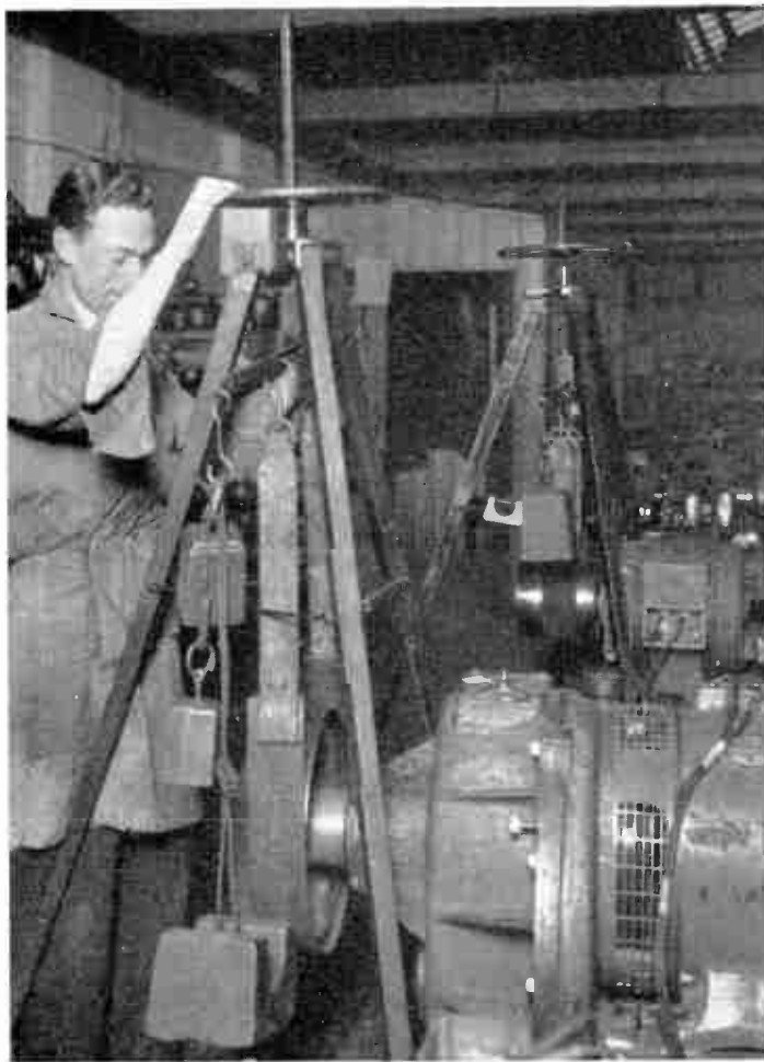
Fig. 13.—BRAKE TEST ON BEARER MOTOR. ( Lancashire Dynamo and Crypto, Ltd. )
