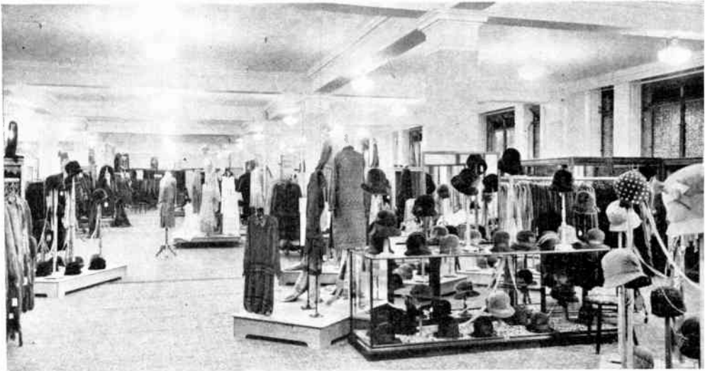
Fig. 1.—How the ENCLOSED DUST-PROOF TYPE OF UNIT IS FITTED IN A LARGE DEPARTMENTAL STORE. It will be seen that the illumination over all is very even and of adequate intensity.
