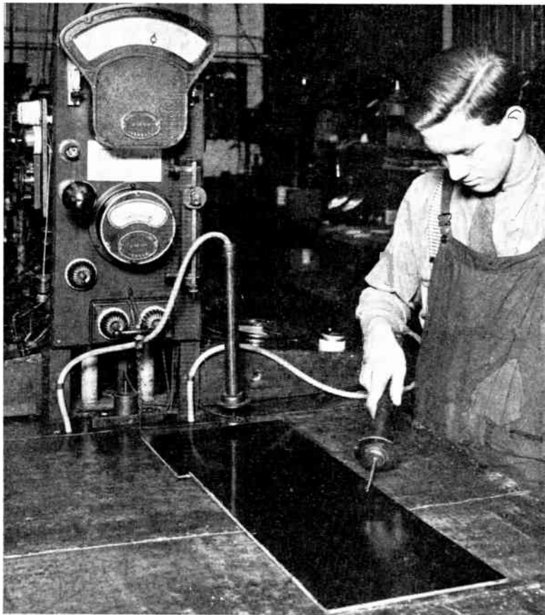
Fig. 3.—TESTING SHEET INSULATING MATERIALS, ETC., FOR DEFECTS.
