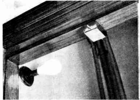
Fig. 3C.—AUTOMATIC DOOR SWITCH IN POSITION.
