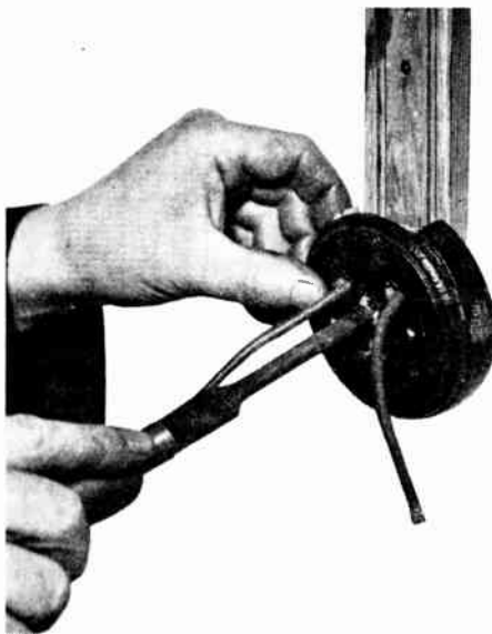
Fig. 42 (Above).—A T BRIDGE CROSSING. The bridge crossing is fitted in the wooden casing system of wiring, to allow wires to be branched away from a main run. The branch wires are looped from a light position on the main run.
