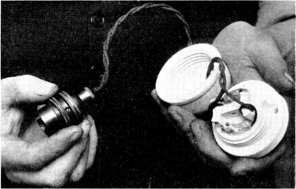
Fig. 4.—A COMPLETE PENDANT WITH CEILING ROSE AND LAMPHOLDER.
