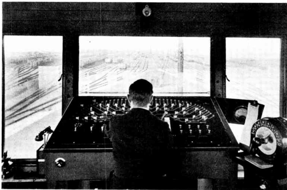
Fig. 1.—THE CONTROLLER AT WORK AT MARCH L.N.E.R. GRAVITY SIDINGS.
