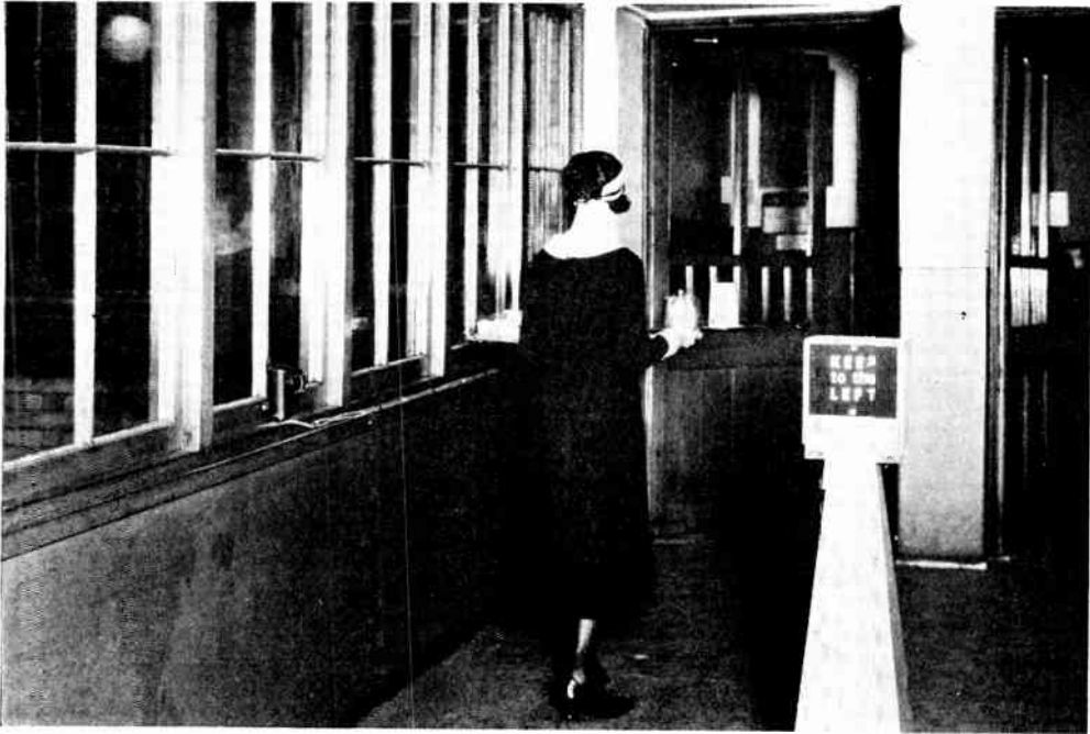
ONE OF THE MANY USEFUL APPLICATIONS OF THE B.T.-H. THRUSTOR MECHANISM. It will be seen that the waitress has interrupted the light beam of the photo-electric thrustor control system and that the door has partly opened. By the time she reaches the door it will be fully opened.
