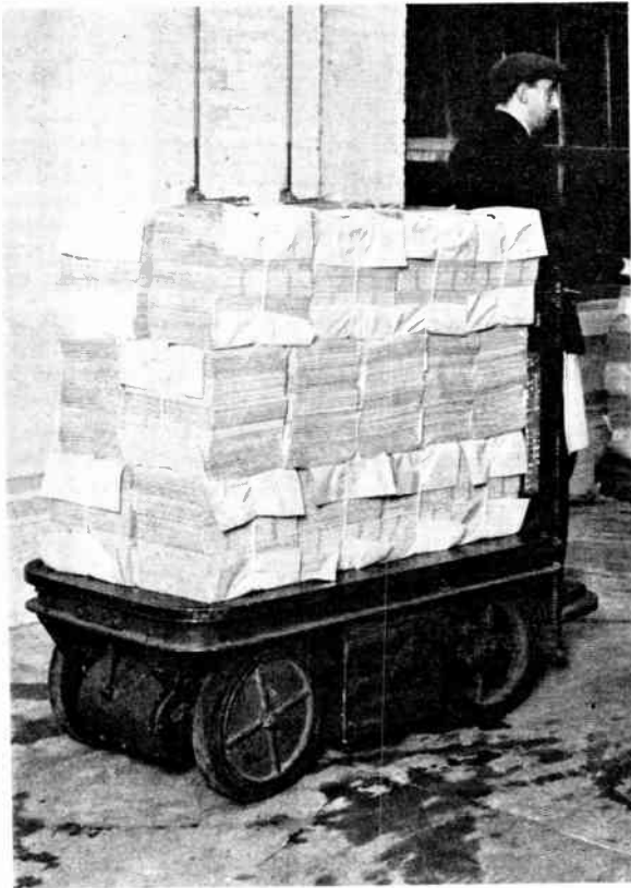
SIX ELECTRICALLY DRIVEN GREENBAT TRUCKS ENABLE THE HUGE OUTPUT TO BE HANDLED QUICKLY AND EFFICIENTLY.
