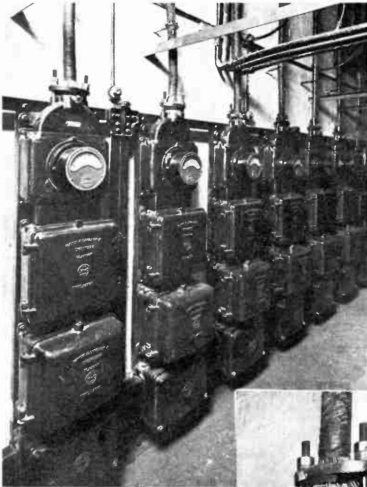
HERE WE SEE THE BANK OF IRONCLAD UNIT TYPE SWITCH PANELS BY M & C SWITCHGEAR, LTD. ON THE RIGHT IS A CLOSE UP VIEW OF GLAND, SHOWING METHOD OF BONDING WIRE ARMOURING
