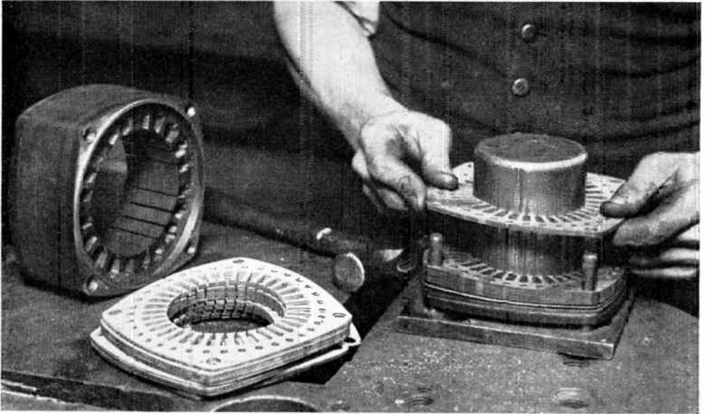
ASSEMBLING THE STATOR STAMPINGS.
