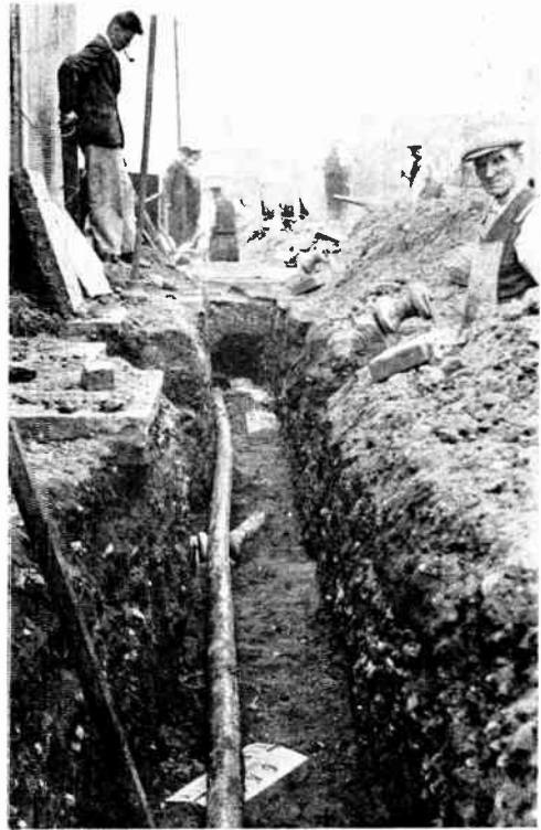
VIEW ALONG CABLE TRENCH. Showing tunnel under entrance to works.
