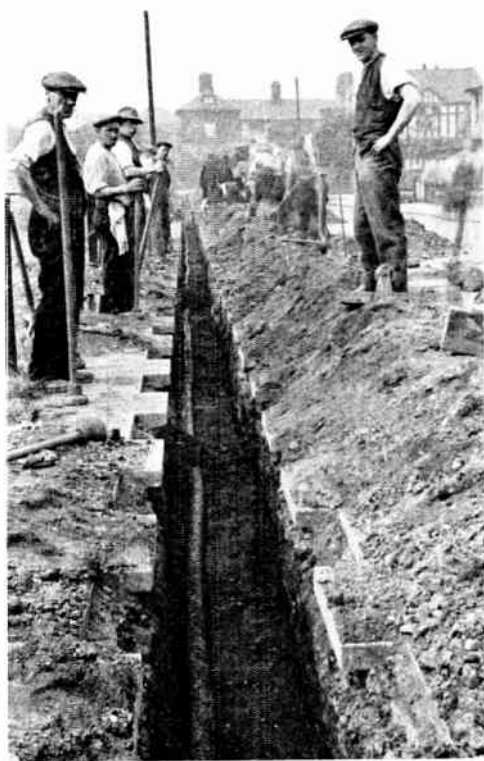
THE CABLE TRENCH BEFORE FILLING IN.
