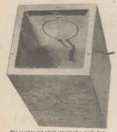
The coupling coil which consists of a single turn of wire is secured to the top of the containing box.
