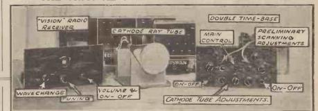
A general view of the first cathode-ray tube receiver used in this country, showing what the various units do and the purposes of the controls. It is interesting to note that this receiver was developed and employed in the "Popular Wireless" Research Laboratories.
