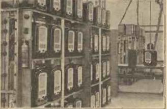
A batch of receivers undergoing a fix hour heat test at the Ferranti works. This is only one of the many tests that Ferranti sets are subjected to before being passed out as O.K.
