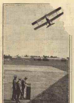
"By simply pressing suitably labelled buttons on a control board the operator is able to make the machine climb, dive or glide, turn to the right or left, and land."
