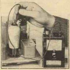
Measuring the anode current of a screen pentode by means of a Pifco Rotameter,
