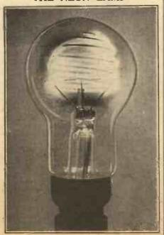
The neon lamp is a practical example of an electron discharge producing a luminous effect.
