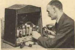
Removing the valves in a superhet so that the circuits can be tested and the valves checked over for characteristics.
