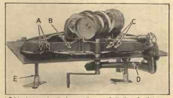
Points where an automatic-changer unit may need attention. See that connections of pick-up at C are tight, that mains contacts at A are secure, that the earth at B is made, that the pick-up adjuster, D, is correctly operating, and that the "lifts," E, are not sticking.
