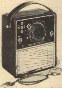
Though not an essential instrument, a calibrated oscillator such as the above is very helpful for such work as condenser ganging.
