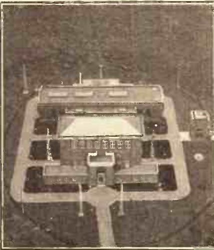
"The transatlantic 'long-wave' telephone uses single sideband transmission." Our photograph shows the station house at Rugby which deals with this class of work.
