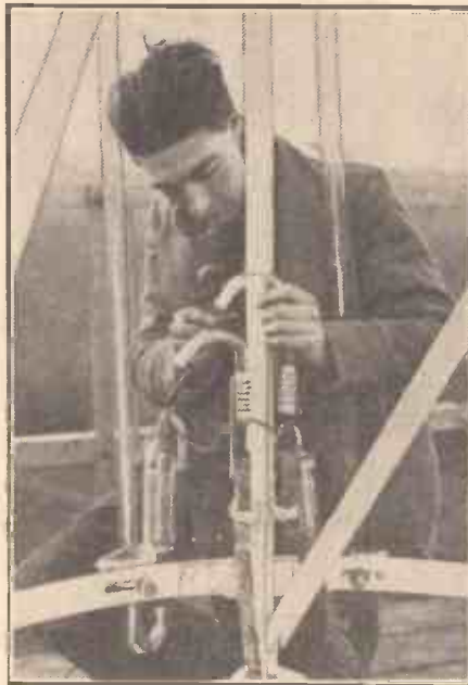
The erection of a neon danger beacon at the Rugby wireless station was begun only a few days before the Imperial Airways liner Apollo flew into a radio pylon at Ruysseide. The Rugby beacon will be visible over a radius of fifty miles.
