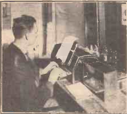
One of the teleprinters installed at the Lympne terminal of the new trans-Channel micro-ray link.
