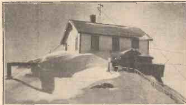
This station, situated at Summit, California, is 7,200 feet above the sea level. It is employed for communication with American air liners, and on account of the heavy winds at this high altitude the building is anchored by steel cables.
