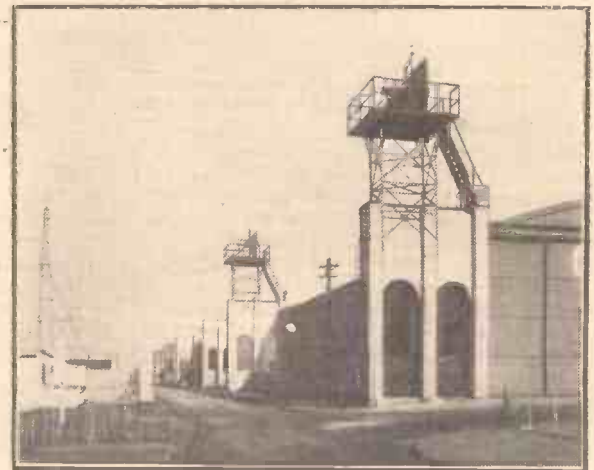
The reflector assemblies and the valve housing are installed on platforms supported by steel towers above the hangars.
