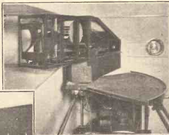
USED BY THE B.B.C. These two photographs show some of the Baird television transmitting apparatus installed by the B.B.C. An engineer is seen making adjustments in the picture to the left. Note that the whole "camera" swivels round on a turntable.
