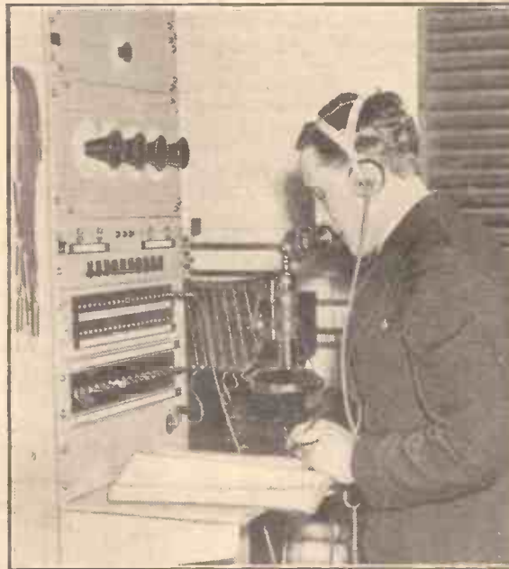
The telephone switchboard at Tatsfield, which is directly linked with Broadcasting House, and to which any of the outputs of the various receivers at Tatsfield can be connected.
