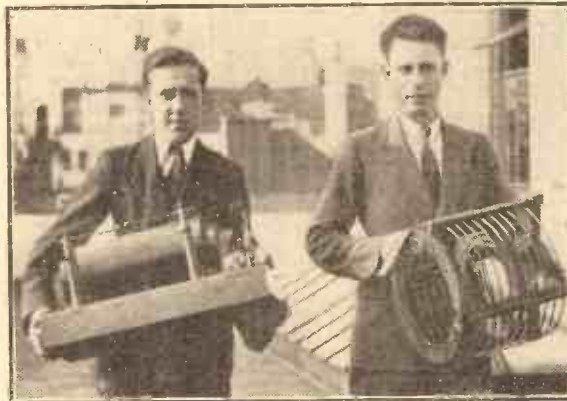
Parts of a spark transmitter that was used in early experiments by Marconi being removed to the new offices of the Marconi Company on the Embankment. They form part of a museum of historical radio apparatus.
