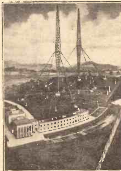
An interesting feature of the station (working on 517 metres) is that one mast only is used for the aerial, the other acting simply as a reflector.
