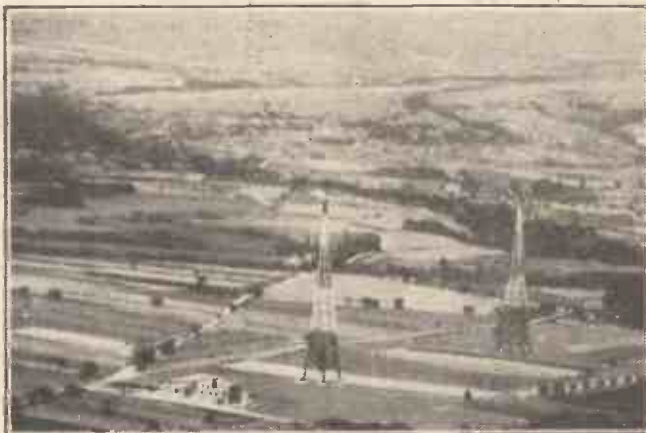
There are a number of different masts and aerials at Prangins, and this view of the two biggest masts was taken from an aeroplane flying on the regular Stuttgart-Geneva route.
