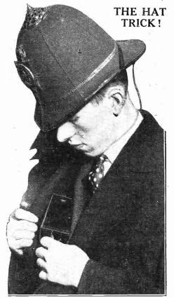
Motor bandits will not approve of this new portable receiver which may be issued to London policemen. By means of a tiny set and cone speaker in the helmet, and a pocket battery, Scotland Yard could keep in touch with any officer on duty.
