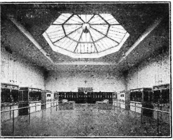
This excellent view of the transmitter hall shows the floodlighting dome; 30 ff: above the ground, which provides all the illumination for tha control, engineers without any glare. The floor is made of compressed cork, a new material for this purpose.
