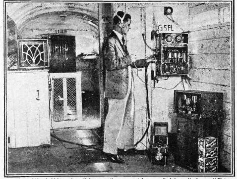
For the first time in history a two-sided conversation was carried on recently between the famous "Flying Scotsman" and the air liner "Heracles" while both of them were travelling at full speed. Here is the compact apparatus which was installed on the train for the experiment.
