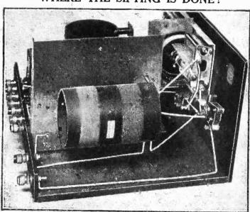
The aerial circuit is tuned by the first coil and condenser, the currents being passed on to the second coil and condenser by the resistance incorporated in the coil unit.
