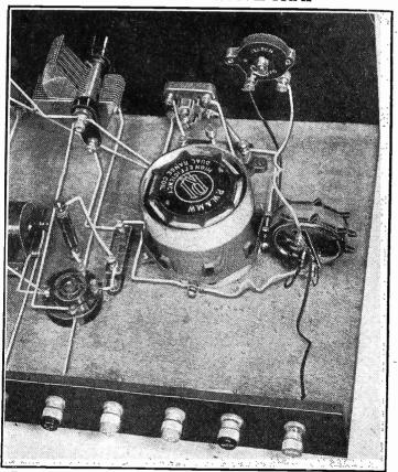
Even if you are unable to "moderate," the Moderator coil and condenser can be used as an efficient wave-trap and for controlling long-wave selectivity, as is explained in the accompanying article. In such a case, however, the Moderator Coil does not have to be placed near any other coil in the set. As shown above it is rather too close to the dual-range coil.
