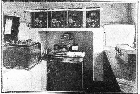
This is a view of the B.B.C.'s own receiving station at Tatsfield, Kent. Here a staff of engineers watches the ether, notes the wave-lengths and any tendency to wobble, and generally keeps a sharp eye on the broadcasting situation.
