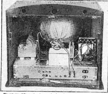
The interior of the receiver is a masterpiece of neat, efficient design. In this photograph you can see the little that can be seen of the actual "works" as the screening is very complete. The three gang condenser and the power transformer however, are visible on either side of the loudspeaker.
