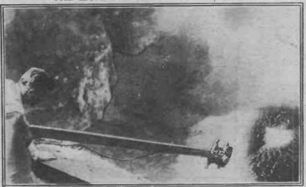
A microphone tied to the end of a long post was used to pick up the noise of a volcano in cruption, for broadcasting via United States stations.
