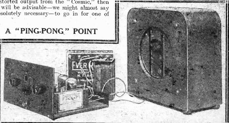
Always strive to avoid facing the loudspeaker towards the set if the two are in close proximity, otherwise the sound-waves impinge upon the valves and are liable to produce annoying "Ping-Pong" noises.
