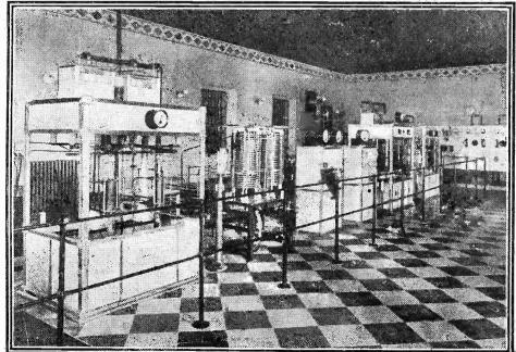
A view of the transmitting gear at the Milan station. With a power of 7 kw., and using a wave-length of 331 metres, Milan works in conjunction with Turin, Genoa and Trieste.
