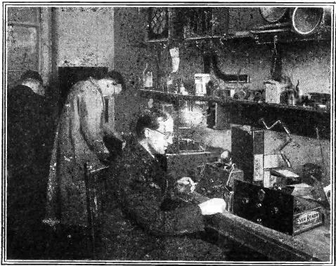
Mr. Dowding testing the "Cosmic" Three, with a valve voltmeter, for sensitivity and selectivity.
