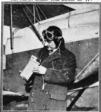
Here is Sir Alan Cobham at Heston Aerodrome inspecting the newly-evolved small radio set for light aeroplanes, which enables the pilot to keep in touch with the ground and obtain weather information and other navigational aids. Heston Aerodrome can often be heard on about 830 metres warning all and sundry of storms to come.
