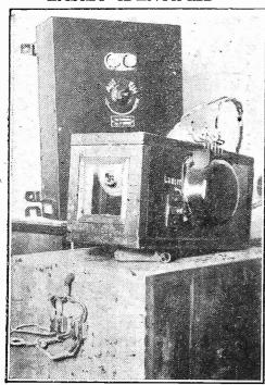
Konigswusterhausen has a metronome interval signal (240 beats per minute). The metronome is kept locked in the bottom lead box, and the microphone can just be seen through the glass side of the box on top.
