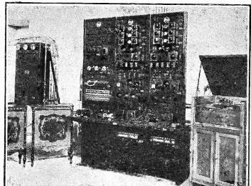
The control panel at the Rome broadcasting station. Rome has a power of 50 kw., operates on a wave-length of 441 metres and has a lady announcer.
