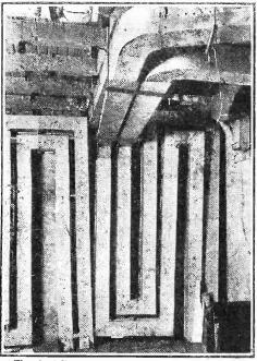
They look like the pipes of a big organ, but actually they are part of the ventilating system at the new B.B.C. H.Q. There are in all approximately 150 tons of ventilating duct in the building.
