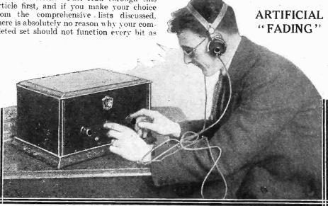
Artificial "fading" effects are very often produced through having the 'phone leads bunched together and resting on part of the body. So when you use 'phones in conjunction with your "Cosmic" for distant short-wave reception, try to avoid the sort of thing illustrated above, and put the 'phone leads as far away from your body as you can.
