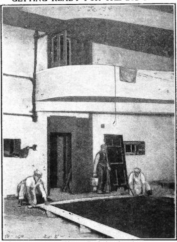
These workmen are engaged in cementing the floor of one of the Broadcasting House studios, ready for the transfer of staff and service from Sayoy Hill.
