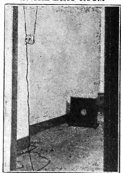
The B.B.C. can add as much echo as it wishes to any studio performance by means of the echo room shown here. It is a bleak and bare apartment, so a speaker's voice, coming from the loudspeaker, "rings" as from a sound-box. The echo-room microphone picks this up, and adds it to the original transmission in any desired degree, the balance between the two microphones being under the control of the engineer in charge.
