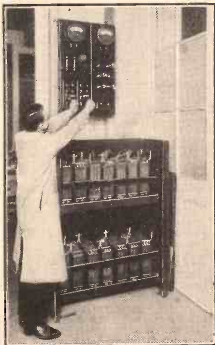
A D.C. system using large accumulators has been installed in "P.W.'s" Research Dept.
