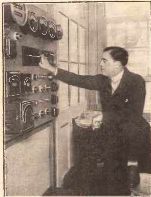
The "P.W." Research Dept. generates its own A.C., and several kw. of A.C. power of any cycles and voltage are always immediately available. The photo shows Capt. Eckersley switching on.
