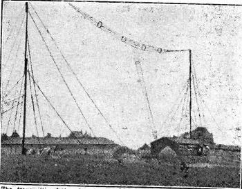
The transmitting hut and aerial of the Dublin broadcasting station. Dublin has a power of 1½ kw., and transmits on a wave-length of 413 metres.
