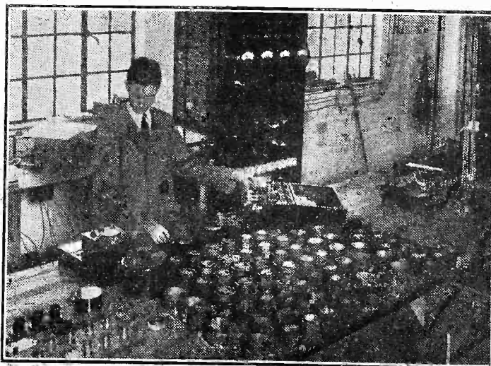
A batch of "P.W." Dual-Range coils being given wave-length tests at the R.I. factory. All the "P.W." coils made by R.I. are tested for inductance and wave-length.
