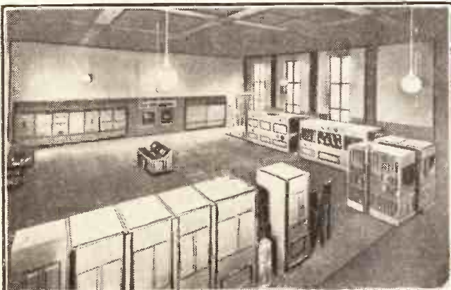
Two views of the 75 kw. plant at Hellsberg—Germany's second high-power station. On the left you see the transmitter hall, and on the right the complicated water-cooling system. The water circulating in the valve jackets is again cooled by other water from outside.
