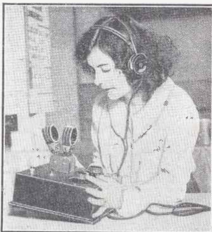
This is a crystal set designed especially for the blind. The dials are calibrated, in wave-lengths, with Braille markings.
