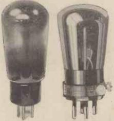
The valve on the left is a Vatea rectifier made by Abbey Radio, and the one on the right a Dario rectifier.
