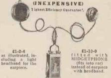
THIS Aid comprises a highly sensitive SUPER-MICROPHONE for taking up Sound (to be attached to Coat or Dress, con veniently concealed), a SMALL BATTERY (for the pocket), and a SMALL EARPIECE which can be held to the deaf ear by hand or by a light headband supplied with the All speech and sound reaching the Super-Microphone is loudly heard in the earpiece. The battery can be switched off when the Aid is not in use.
