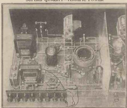
Here is the low-frequency end of the set, which takes the clean, strong signals given to it by the detector and builds them up to really impressive loud-speaker volume. Note the simple and direct wiring.
