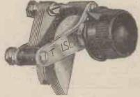
Telsen Variable Condensers (Bakelite Di-electric). Particularly designed for use as a reaction condenser, may also be used as a neutralising condenser where large capacity
