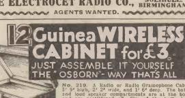
No. 219. A Radio or Radio Gramophone Cabinet, 5'9' high, 2'2' wide, and 1'6' deep. The battery and loud speaker compartments are at the bottom and are partitioned off. Size of the bafflo behind the fret is 24' x 24'. Metallio fabric for the fret front is included. Opening at the top and back. This cabinet will take a panel 2' x 9' or smaller.
