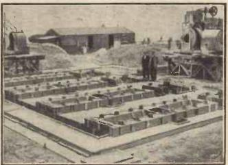
Rapid progress is now being made at Moorside Edge in the building of the new North Regional station. Here you see the 600-ton concrete bed for the engine-room.
