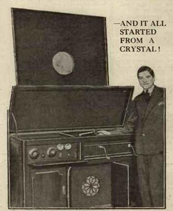
Six years ago, when at school, he made a crystal set, and then he got "valve fever" and made bigger and bigger sets, giving more and more volume. This outfit is a seven-valve Radiogram receiver, with two double-spring motors, and two 12-inch turntables. The volume of sound is said to be "equal to three bands"—and yet it was a spare-time job!
