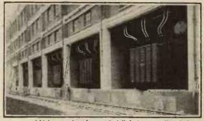
by the Ferranti people. Transformers installed at a generating station by the Ferranti people. Transformers such as these have to handle colossal amounts of electrical energy, and very special precaution have to be paid to the dissipation of heat.
