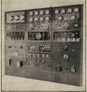
This is the crystal control panel at the new 50 kw. broadcasting station at Rome, which can easily be picked up in this country on 441 metres. (It calls "Radio-Roma.") The crystal control keeps the wave-length very steady, and prevents "wandering."
