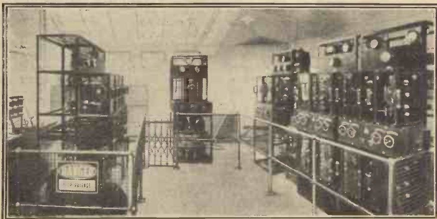
The Marconi 12 kw. broadcasting transmitter at the London Station. There are six panels, and from left to right they are: Two rectifier panels, one independent drive panel (centre), one main oscillator panel, and two modulator panels.
