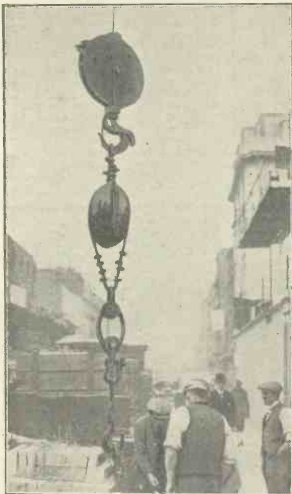
A crane working near the London broadcasting station becomes strongly charged up by the energy transmitted, and workmen have received shocks when handling the bucket. To prevent this, the large "egg" type insulator shown above has been inserted.
