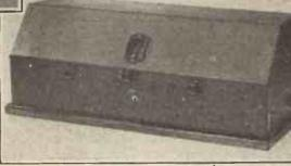
A popular model of the hornless loud speaker is shown to the left. (Note how the centre of gravity has been placed over the base to give the instrument stability.)
