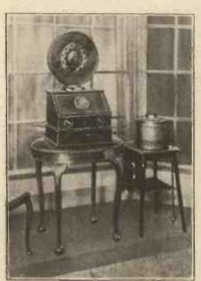
Some magnificent sets and associated equipment are to be seen at the numerous stands occupied by the Marcomphone Co., Ltd. Above, one of their sets is shown above connected to a thermopile. This enables L.T. to be derived from a gas supply. The assembly was exhibited last year.
