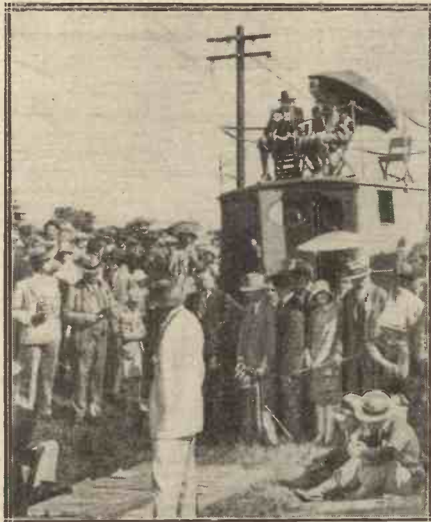
The modern commentator is greatly assisted by the special new B.B.C. van, shown in action herewith. The roof of the van serves as an observation studio, and in the interior are all the necessary amplifiers and so on.
