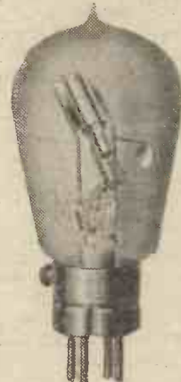
The K.L.1—the first British A.C. valve.
