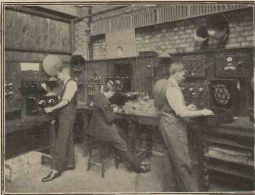
This is a corner of a testing-room in a large radio factory, and the men are busily engaged in thoroughly checking the capabilities of the finished receivers. In the centre can be seen a device used for testing the quality of reproduction of electric gramophone sound boxes and their associated equipment. (Burndept Wireless, Ltd.)
