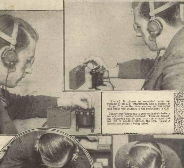
The test made with a battery and 'phones connected in series can be applied not only to one coil or winding, but to a whole scheme of connections.
