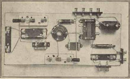
Portion of the apparatus employed by Mr. Harris in testing components. In this case a valve detector passes its rectified current through the primary of a telephone transformer, and the current in the secondary is rectified by a crystal and finally passed to a microammeter.
