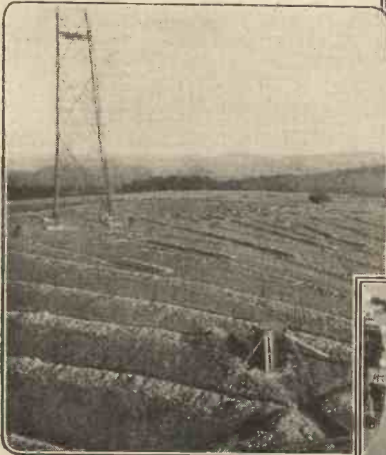
(Above) Thick wires are buried in the above trenches. These form the extensive "earth" which covers a very large area. The base of one of the masts is also shown.
