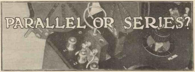
THE easiest way of explaining the meanings of the terms series and parallel to anyone not too well acquainted with the principles of electricity is as follows: Two components connected up in series are so joined together that the current flows through each one in turn; when two components are connected in
