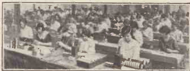
Assembling the new Igranic triple honeycomb coils at the Bedford Factory.
