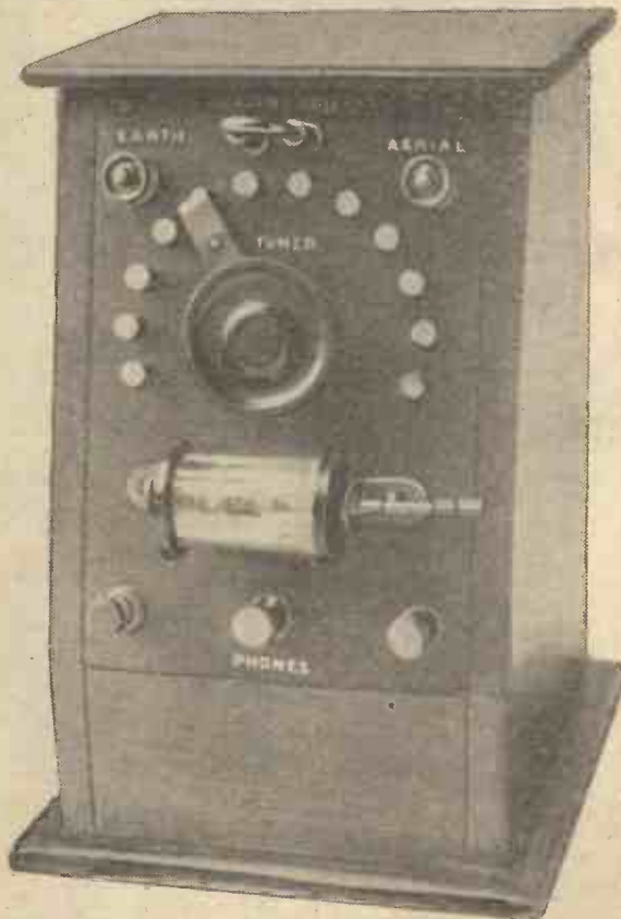
An efficient crystal set constructed by Mr. F. J. Griffin, Lloyd's Bank House Kineton, Warwickshire.
