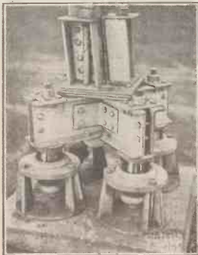
The foot of one of the masts of the new American 50 kw. broadcasting station which operates on 455 metres.
