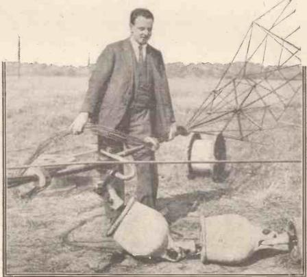
Erecting one of the aerials at the new Rugby Station. Note the huge insulators and heavy aerial wire.
