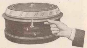
Fig. 2. A "No-dial" Receiver, which contains 5 valves, and is tuned by rotating the lid.
