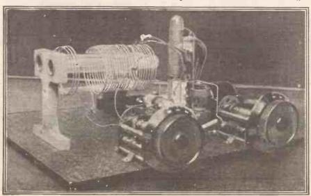
The two slow-motion condensers and the coil-holder are clearly seen in the above photograph, with the choke fixed vertically to the right of the coils.
