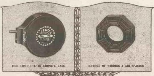
The Windings of the SLEKTUN INDUCTANCE COIL are spaced and separated in the most scientific manner, giving the Lowest Distributed Capacity with High Inductance.
