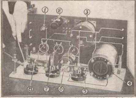
Soldering one of the filament leads. The figures on the photograph denote the following: (1) L.T. switch; (2) L.F. choke; (3) A.T.C.; (4) R.I. tuner; (5) grid leak and condenser; (6) Eureka grand transformer; (7) 1 mfd. condenser; (8) second stage transformer.
