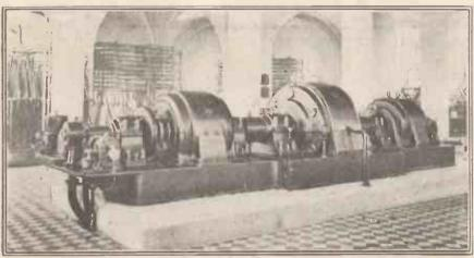
The H.F. alternator (500 kw.) at the St. Assise wireless station, near Paris.
