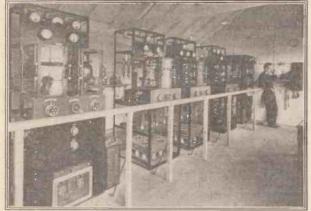
The 6 kw. Transmitter at the Belfast Station.
