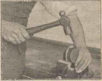
Fig. 3. Bending the contact switch back plate.
