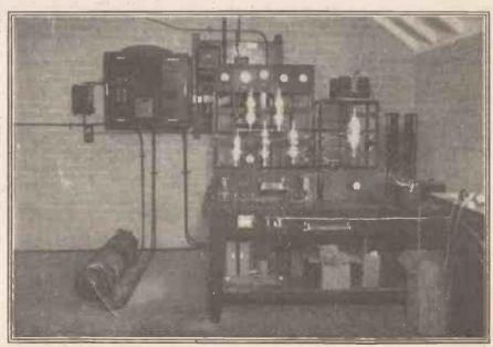
The transmitter, modulating panel, switchboard and generator, at the Stoke-on-Trent relay station.
