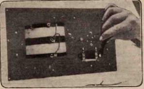
Fig. 6. The grid leak and condenser in position.
