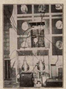
Part of the transmitting apparatus, showing the A.T.L and two power valves.
