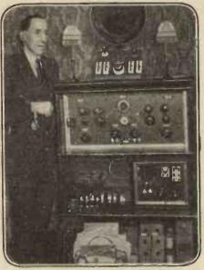
A typical amateur receiving station assembled specifically for loud speaker work.
