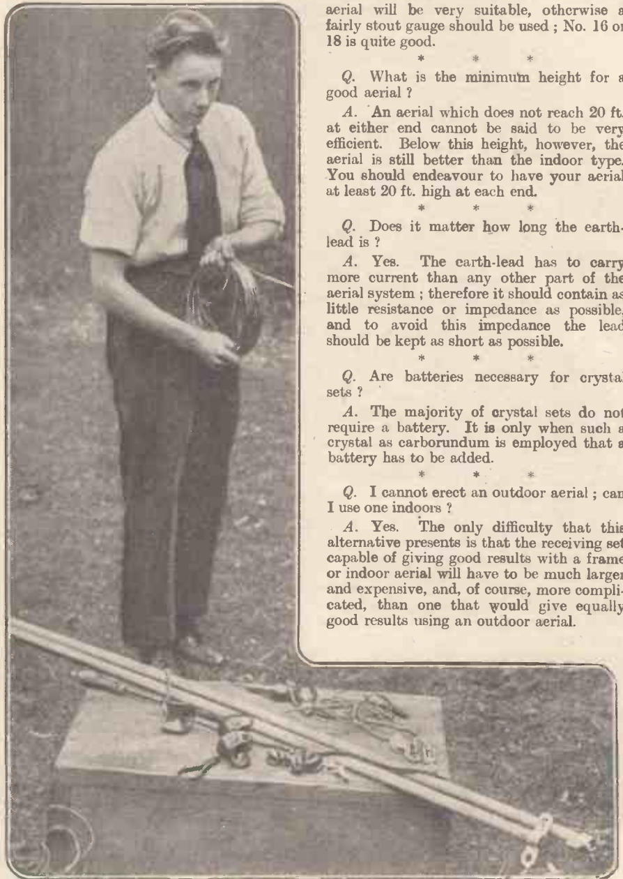
An aerial outfit, showing spreaders, insulators and wire.
