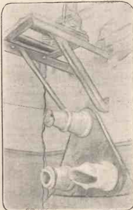
Smashed insulators and aerial switch at the Turkish station, Bagdad, 1917.
