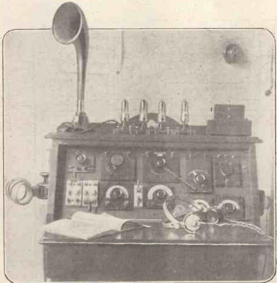
A 4-valve receiving set built into a small writing bureau by Mr. R. C. Common, 74, Murray Place, Stirling.
